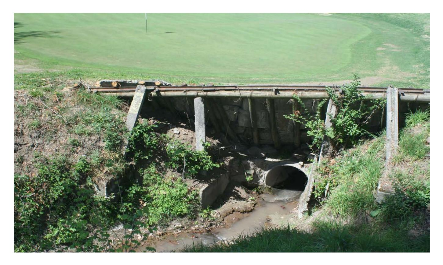
At present the entrance to the pipe going behind the green is very susceptible to erosion, and could in the case of a really bad flash storm, take out part of the green. Also to note from the angle of the pipe we don't think that the pipe goes under the green, which could leave some options regarding the reduction of the break on the green.
