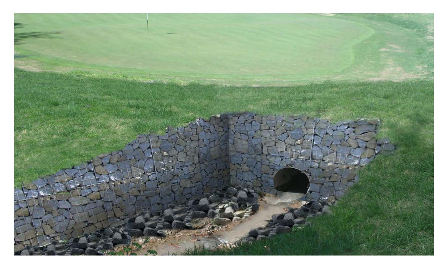
We propose to protect the entrance to the pipe with gabions, which shall protect the green in case of a severe flash storm.
